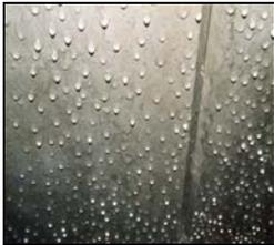
**1) Humidity of indoor air:** Condensation appears when the indoor air in a room cannot hold the level of moisture. Warm air can hold more moisture than cold air. For example, running a bath causes steam. As the air in the bathroom fills up with water vapour, it can no longer hold all the moisture that it contains. As a result, tiny drops of water appear, and develop first on cold surfaces such as mirrors and window sills.
